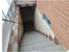
Pic. 3: Basement entrance
